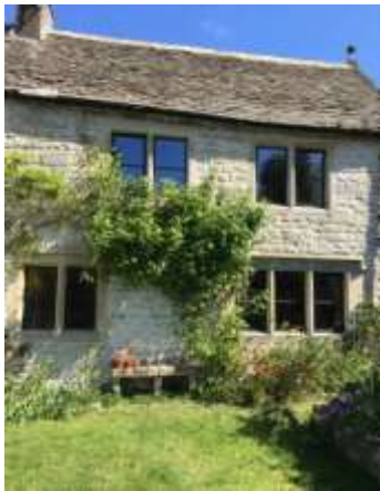
Original draughty metal casements replaced with appropriate metal double glazing
