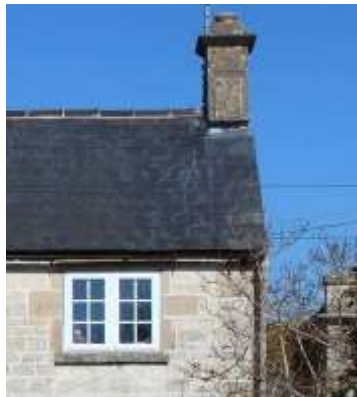
Slate roof on 19 century cottage with a coursed ashlar window
