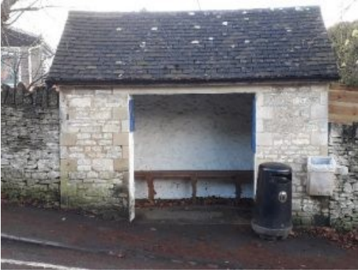
Bus shelter prior to a refurb
