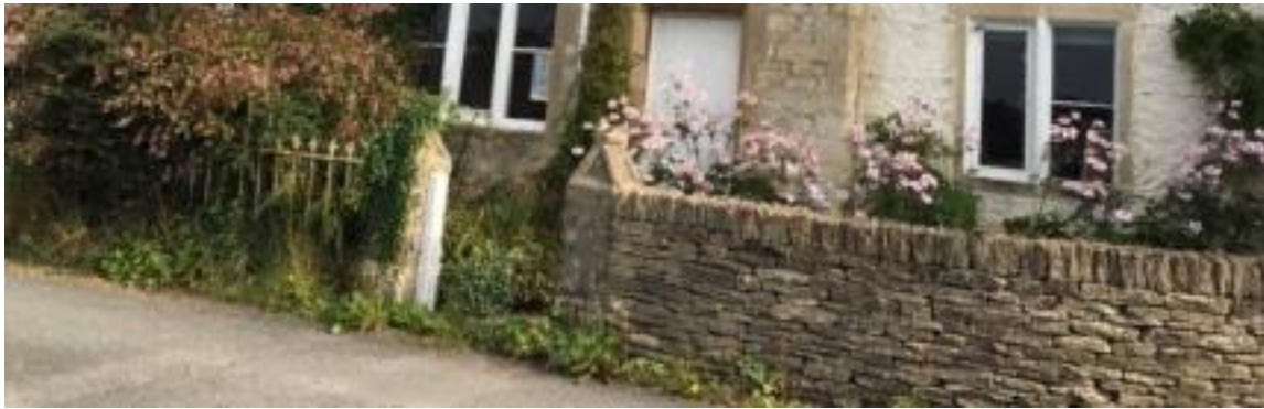
Railings set into a low stone wall, Victorian gateposts and stone wall with vertical stone coping. A rare example, with others in Dr Crouches Road.
