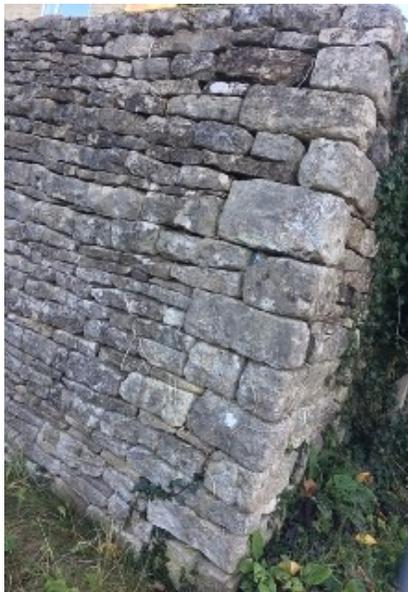
← Retaining wall with stone quoins with narrow layers of brash and flat stone capping.
