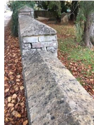
Typical and well constructed stone wall showing stepped design and curved wall. Note the fine gate post. One of the best examples of stone walling in Eastcombe, and by Henry Hook's company.
